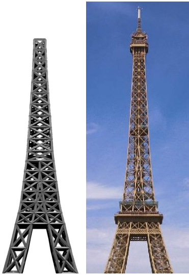
Figure 9: Our trusswork tower, compared with a detail of the Eiffel Tower. Because they are ornamental and not structural, the observation decks are not included in our tower.
